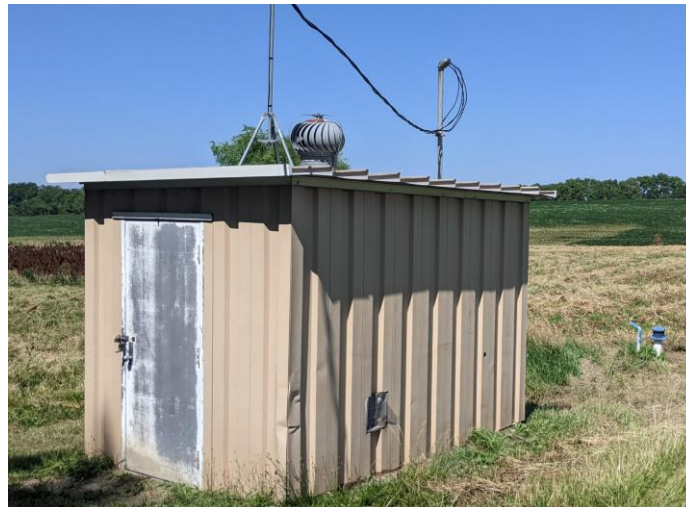
Figure 2; Above-Ground Metering and Control Structure
