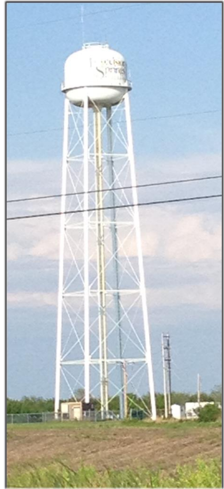
Figure 8: Legged Tank Example
