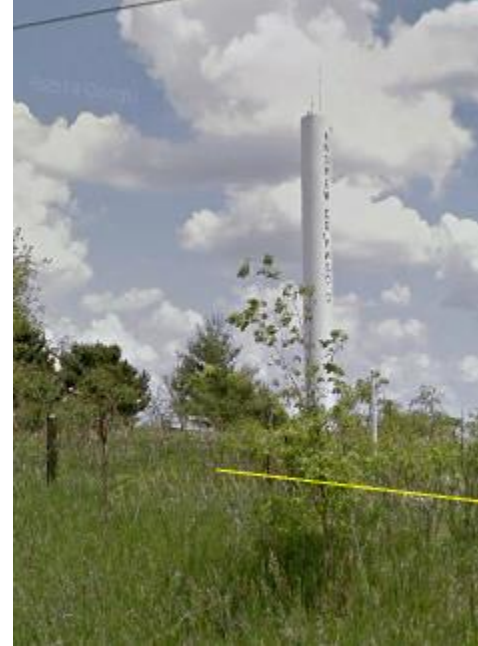
Figure 9; Existing PWSD #3 Unused Standpipe
