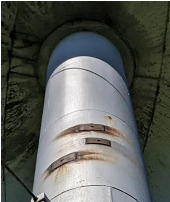
Figure 3; Existing Wet Riser Spot Repairs
